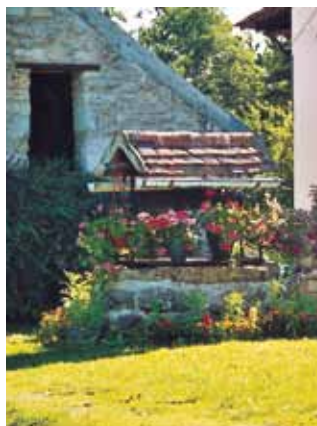
Puits "trop chargé"
