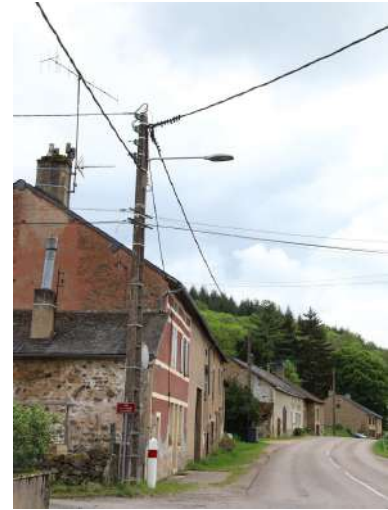
Photos : Renovation of HPS lights by LED - 2 400 K (source : Emmanuel Clerc)
